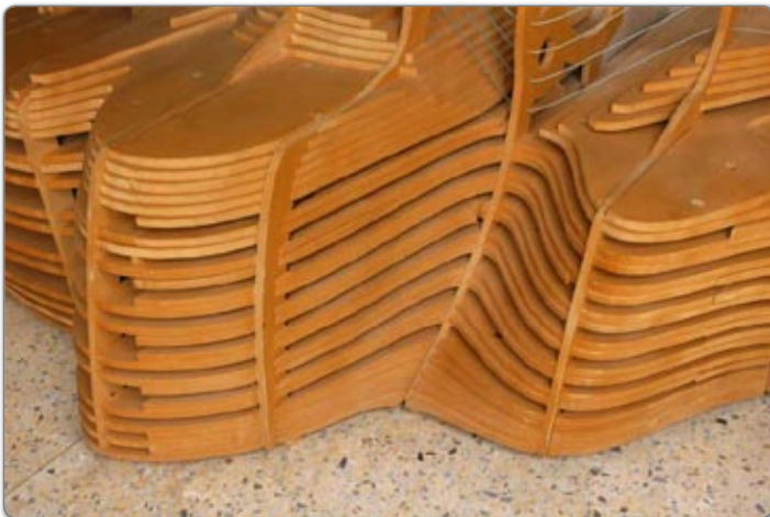
Figure 6: The continuous base stacked up with staggered boards.
